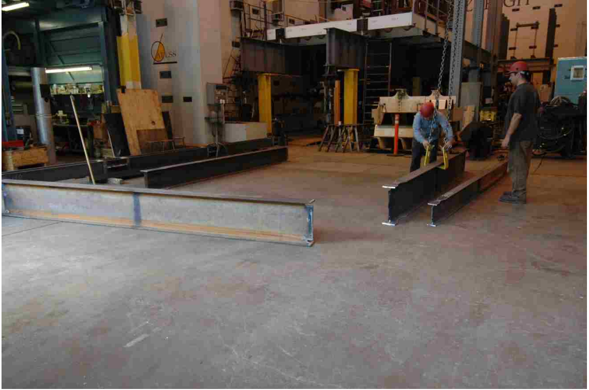
Figure 4.11 – MRF Being Assembled
